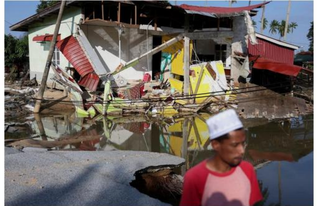
A house that was partially destroyed after flood waters swept through Tumpat district in Kelantan, Malaysia. PHOTO: REUTERS
